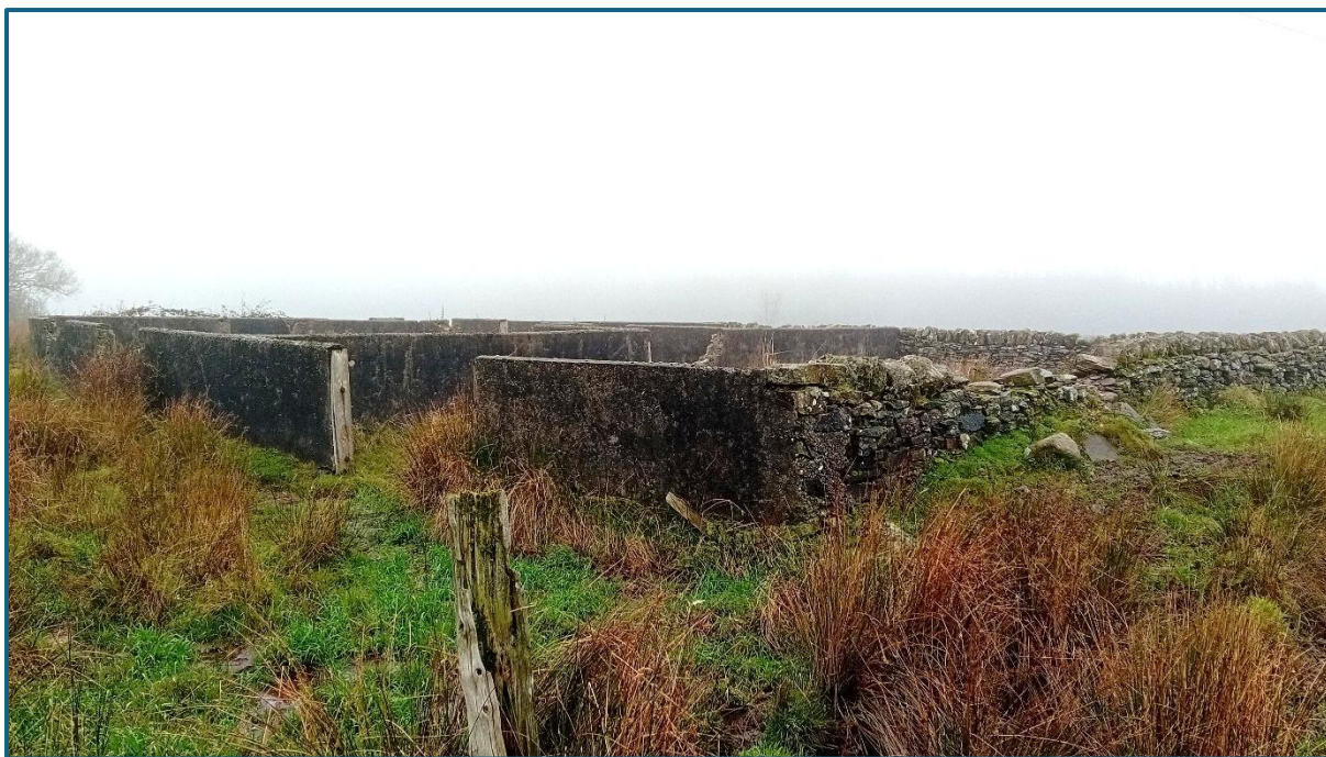
Plate 9 – View of Asset 113 (looking northwest).
