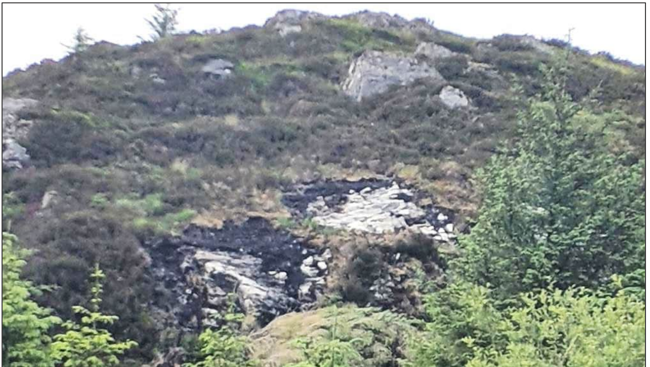
Photo A10.4.4: Localised soil slide and erosion noted 150 m south from proposed T10
